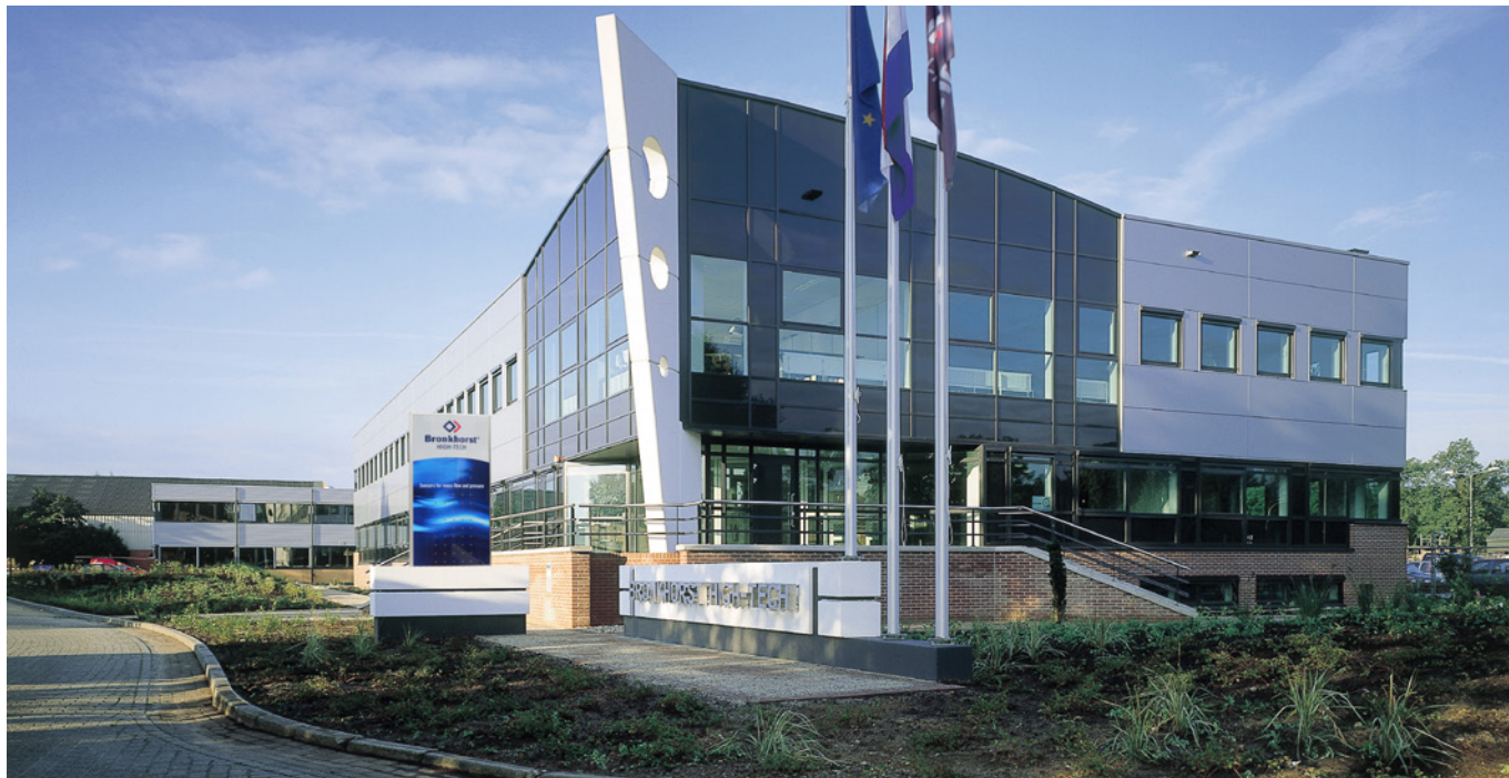
BRONKHORST HIGH-TECH HEADQUARTERS, THE NETHERLANDS
